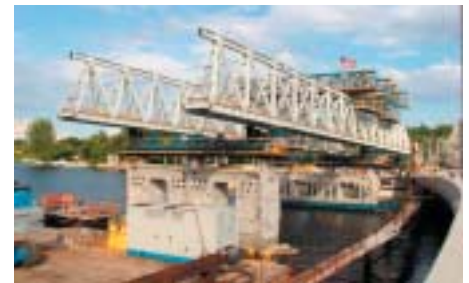
▲ Precast segment floated into position on a barge.
